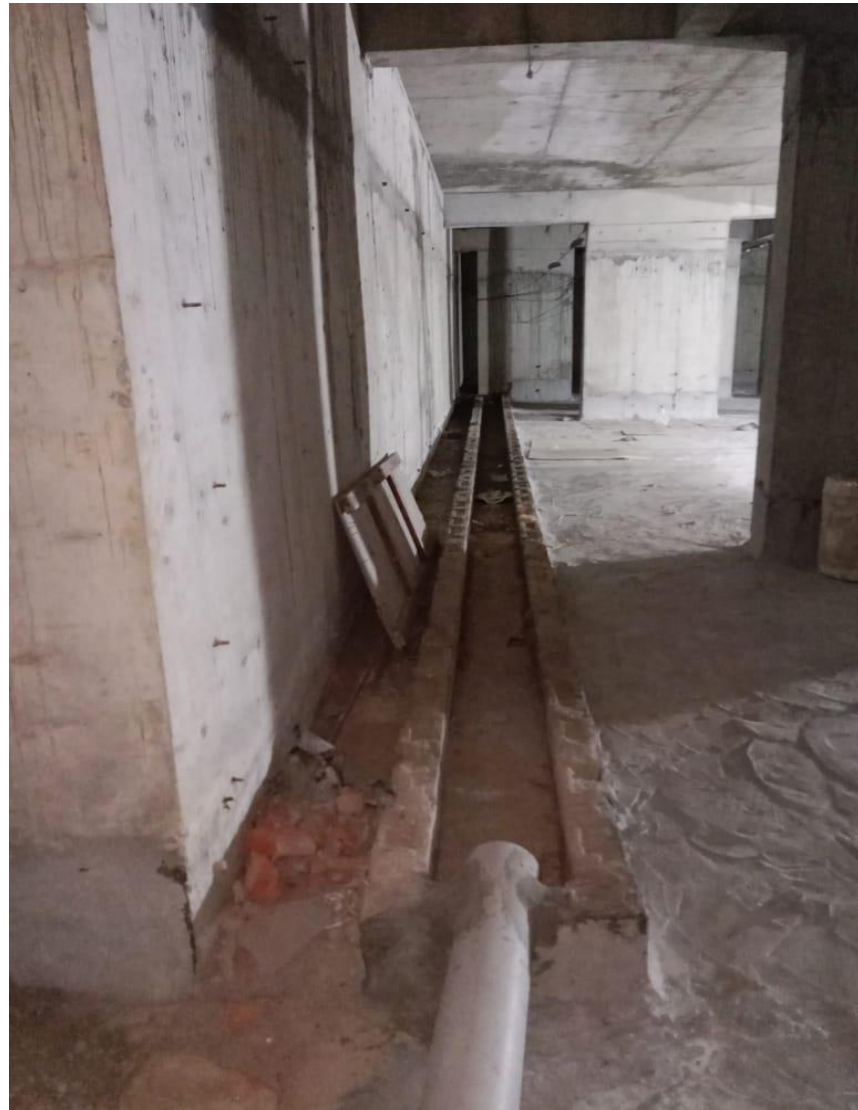
Basement: Drainage Work
